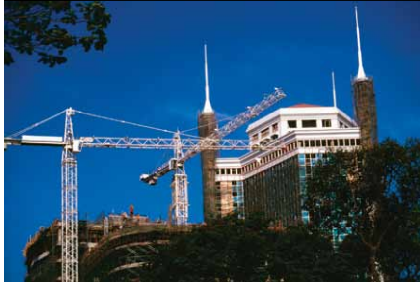
A high-rise under construction in Ho Chi Minh City, Vietnam.
