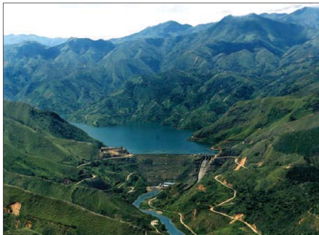
Salvajina reservoir and hydroelectric center operated by EPSA.
