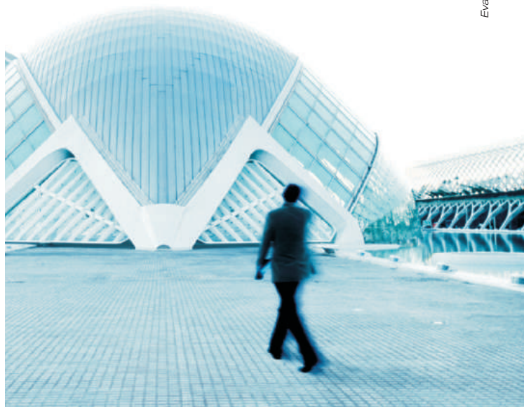
Spain strides towards the future: Santiago Calatrava's City of Arts and Sciences in Valencia
